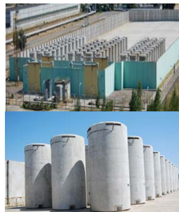
Fig. 6. The dry spent nuclear fuel storage site
